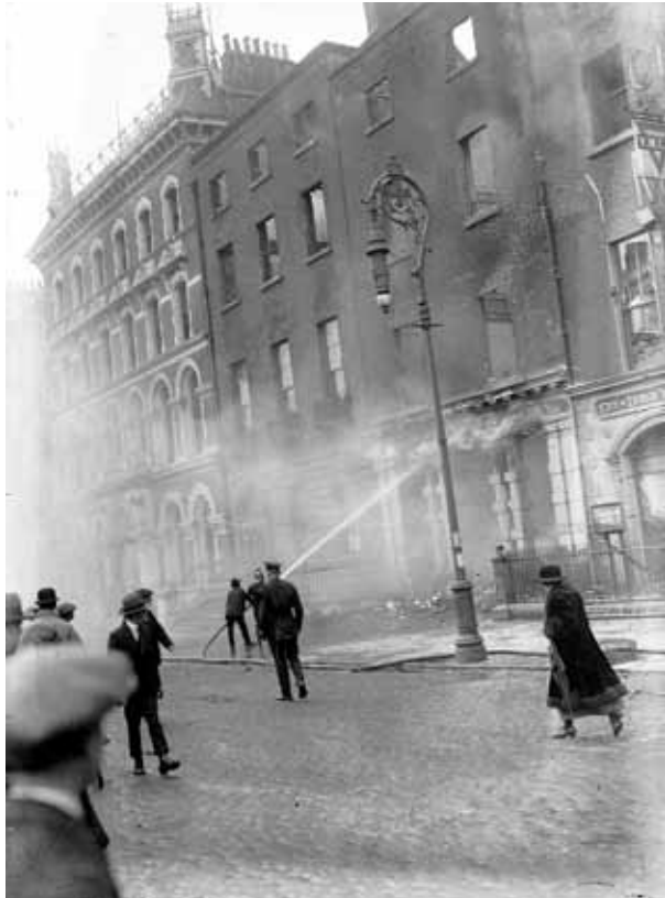
The YMCA and other buildings on fire. (Courtesy of the National Library of Ireland)
